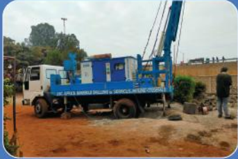
Mashimoni bore drilling in progress
