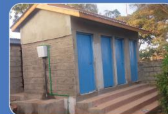
New toilets constructed
