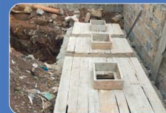
Water reticulation system to recycle waste water
