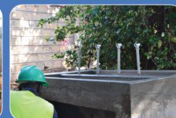
Handwashing section under construction
