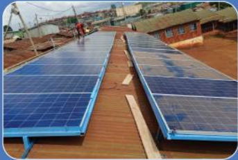
Boreholes solarized to reduce operational costs
